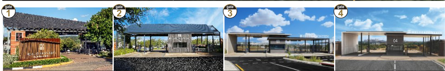
4x Secure Estate Gate Houses, manned 24/7
